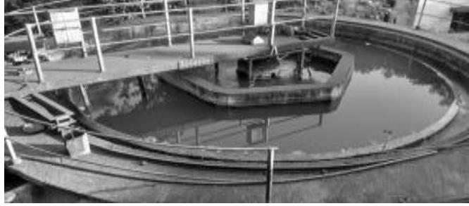
Fig 4: Mechanical Flocculator
