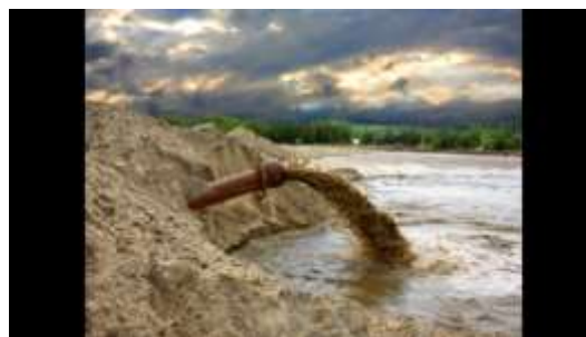
Fig 15: Mine Water Discharge Collected in the Small Pond
