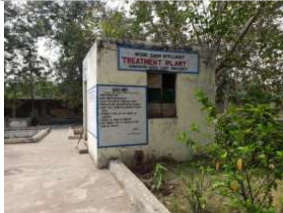
Fig 9: Front View of W.E.T.P (Durgapur OC, Chandrapur Area)
